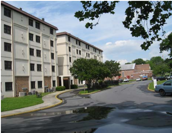
Housing Authority High-Rise
