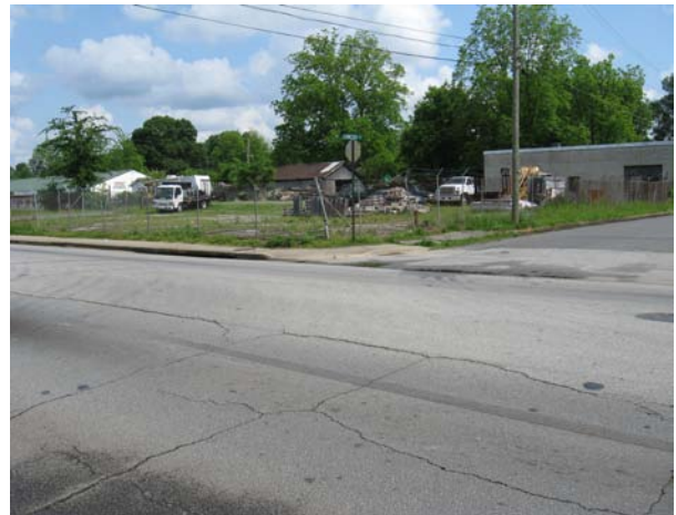
Dilapidated Commercial Area
